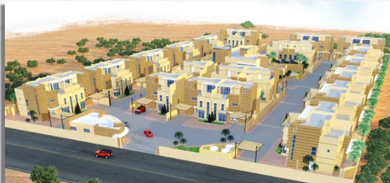
34 VILLA COMPLEX Muraikh
