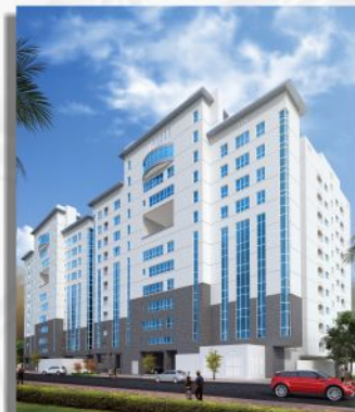
B+G+10 + P APARTMENT BUILDING Musheireb
